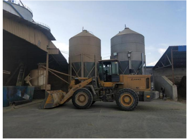
粉状饲料储罐
